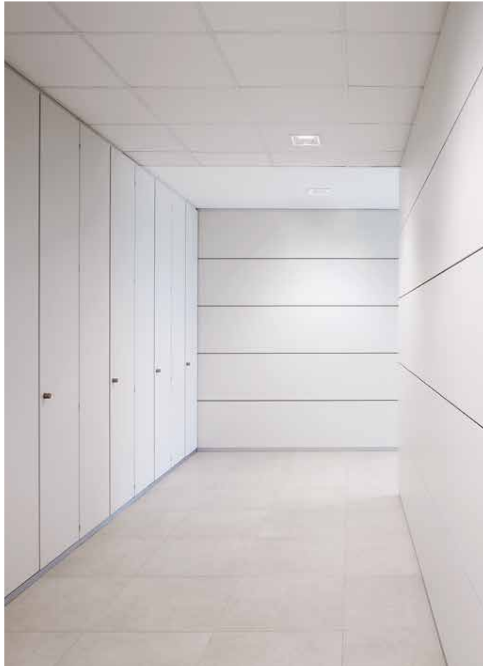
parete Vision cieca a fasce orizzontali/ Vision solid partition wall with horizontal modules
