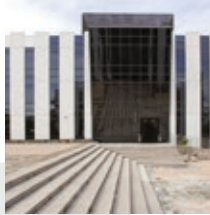
MADRID GLOBOMEDIA PROJECT BY BNB PROJECT
